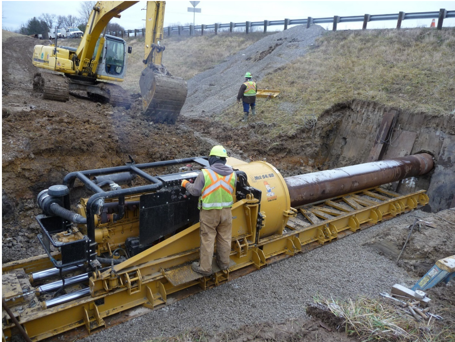
Fig. 1. Setup of the auger boring machine.
