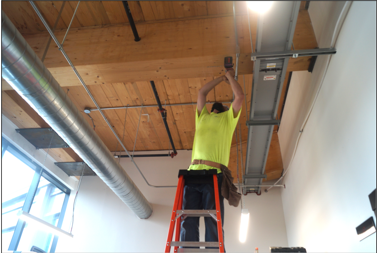
Figure 4. Foreman installing \frac{3}{8} " fasteners into the bottom on the mass-timber beam.
