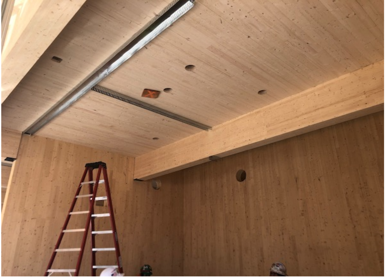
Figure 1. CLT Ceiling panel with pre-drilled penetrations
