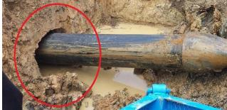
Figure 4. Overcut created by folded CMP
